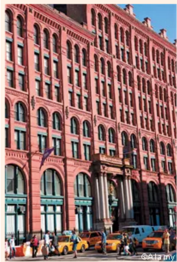
The Puck Building in downtown Manhattan, where there are plans to develop six high-end penthouses, rumoured to cost between $15m and $50m each
